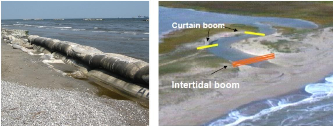
Figure 1. Sand bags deployed at the waterline: an overwash protection strategy
