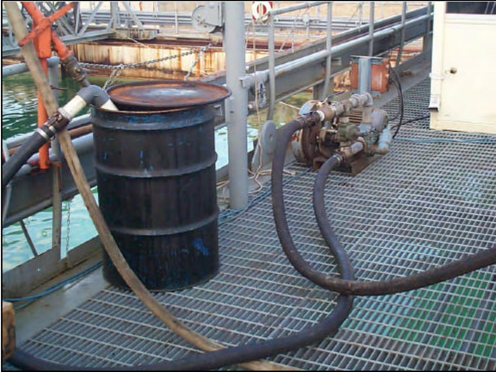
Figure 6. Oil Delivery Pump and Supply Drum
