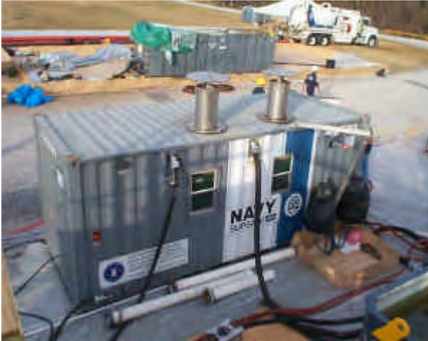
**Figure 8. The U.S. Navy Steam Generator. This provided steam supply for water lubrication and steam coil devices.**
