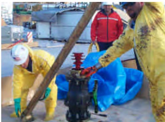
Figure 18. Loading the Scraper Pig
