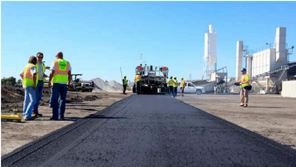
Figure 5 Test plot of asphalt being installed during proof-of-concept test
