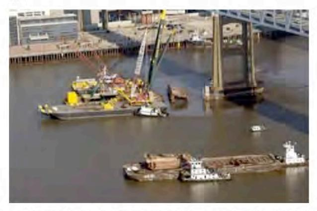
Another major part of the oil spill response was the lightering and salvage of the barge. Each end of the barge had to be secured before lightering. For the bow section, pad-eyes had to be fabricated and welded-on so a crane could partially lift the bow section, to keep it from moving, while divers tapped into the tanks. For the aft section, lifting straps had to be slung underneath
